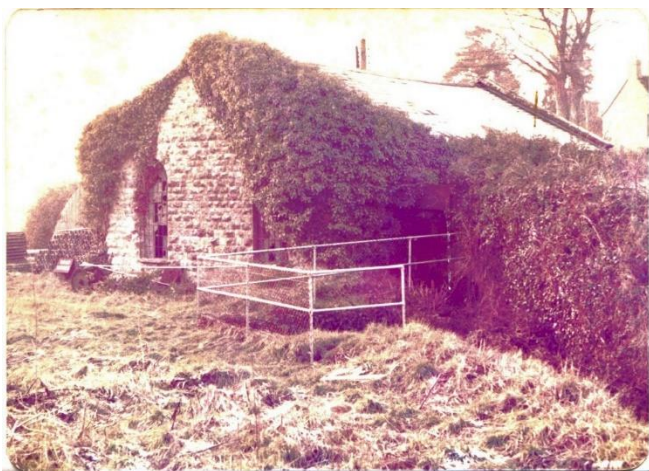
The pump house before restoration
